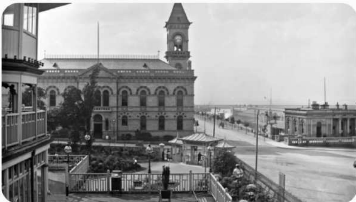
The original roof of the Kingstown station can be seen on the right of this photo to the rear of the station building. Picture courtesy of National Library of Ireland
